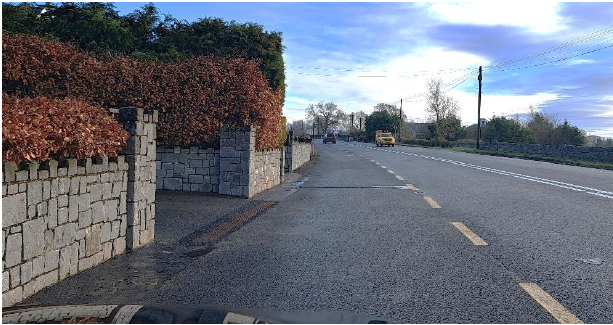
DRAINAGE REPAIR WORKS RECENTLY COMPLETED ON THE R446 AT MACKNEY, BALLINASLOE
