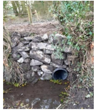
ROAD DRAINAGE WORKS AT ALLINTUBBER/NEW INN TO REMOVE FLOODING FROM ROAD
