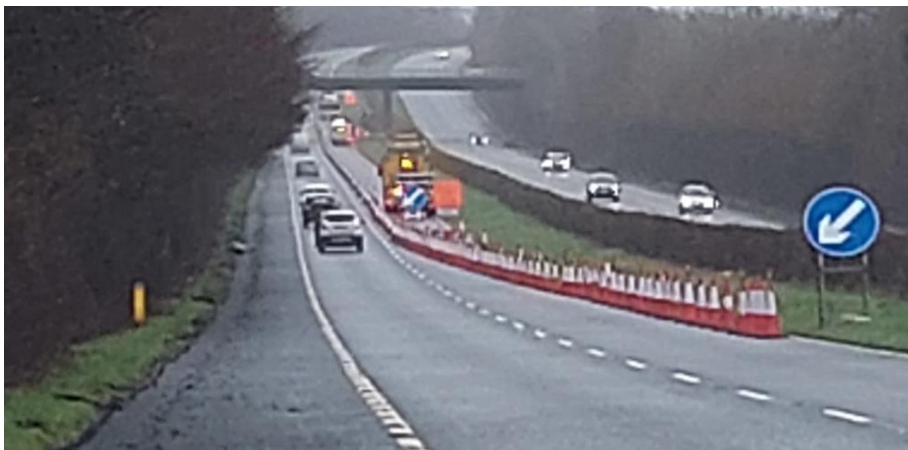
DUAL CARRIAGEWAY SAFETY BARRIER REPAIR
