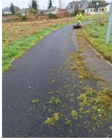
WALKWAY MAINTENANCE WORKS AT CORRY'S FIELD, LOUGHREA
