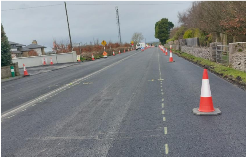
ROAUNMORE - OVERLAY WORKS
