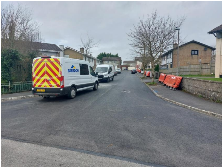
NEW SURFACE INLAY COMPLETED AT COSCORRIG VIEW, LOUGHREA
