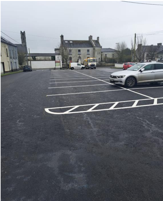
RESURFACING OF EYRECOURT CARPARK
